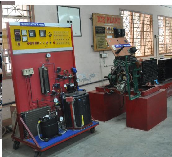
Refrigeration and Air Conditioning Lab
