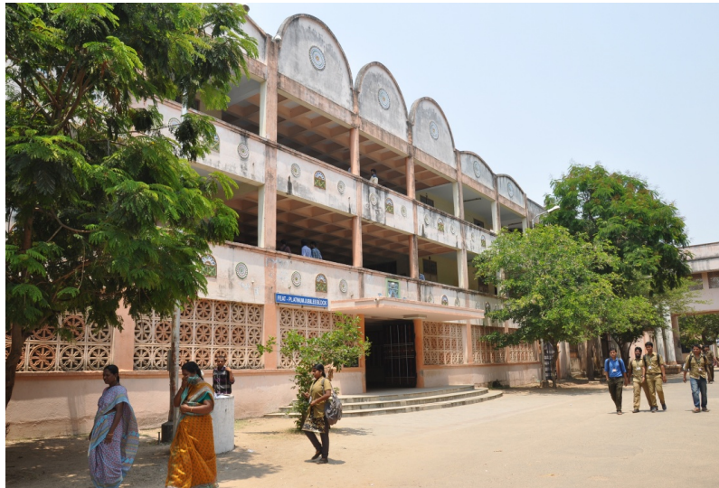
Class Rooms Platinum Jubilee Block
