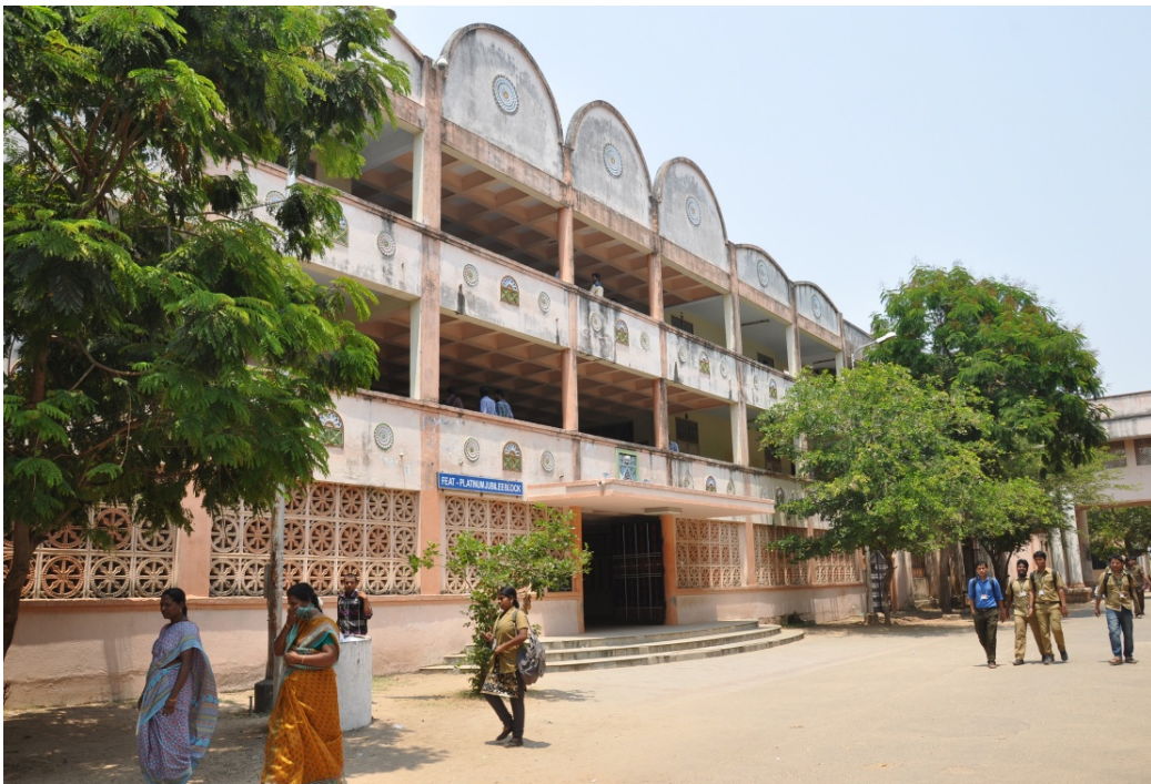
Class Rooms Platinum Jubilee Block
