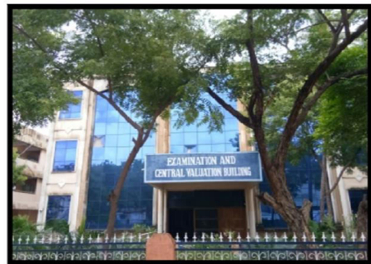
Examination and Central valuation Building
