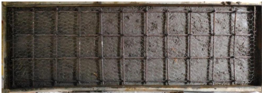
Fig.13 Placing of Skeletal Steel
