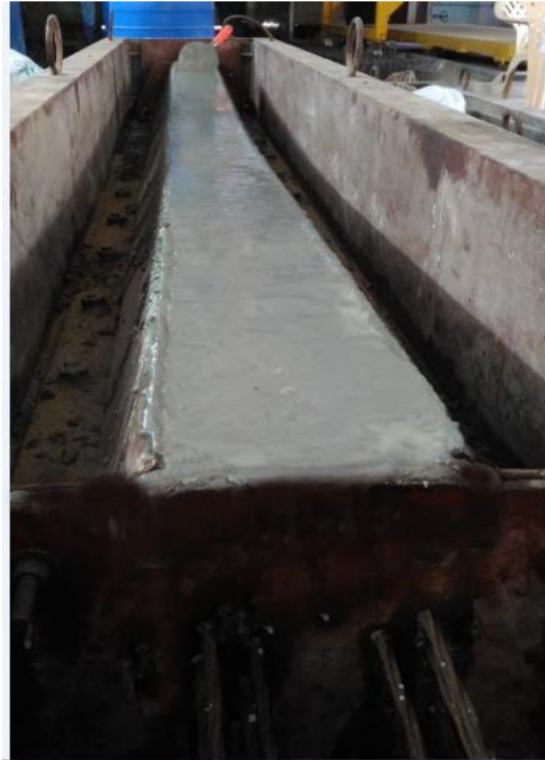
Fig.5 Casting of OPC Sleeper
