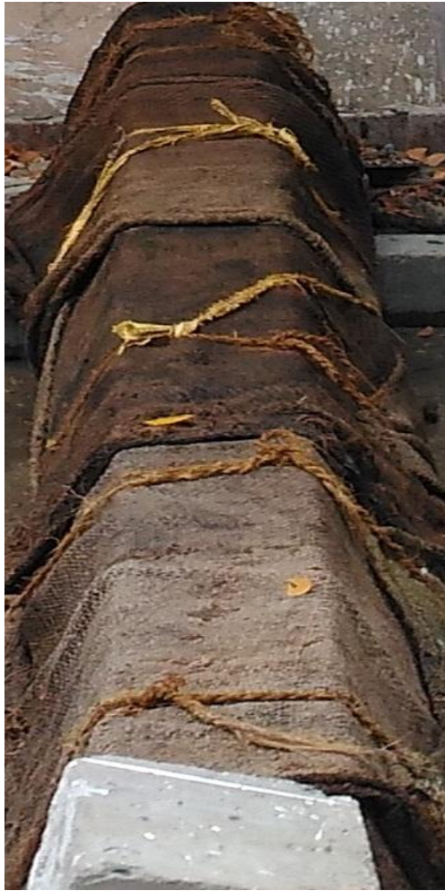
Fig.7 Curing of OPC Sleeper
