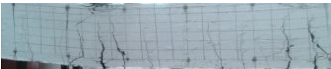
Fig.8 Crack Pattern of GB1
