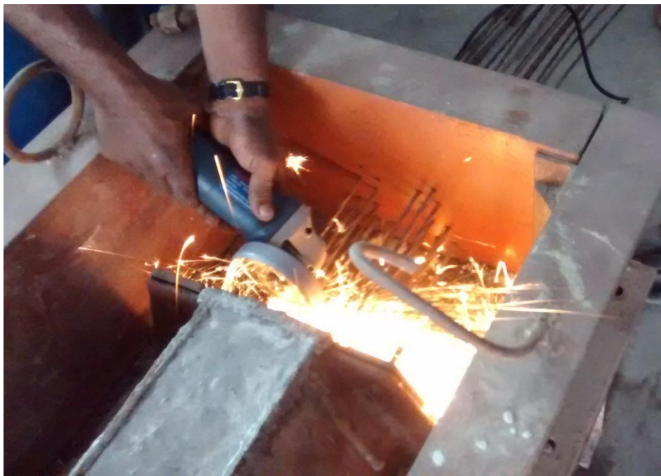
Fig.6 De Tensioning of Strands
