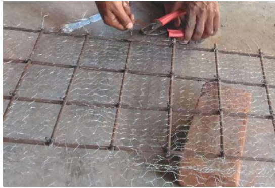
Fig.6 Tying of Meshes
