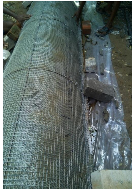
Fig.2 Reinforcement cage on mould
