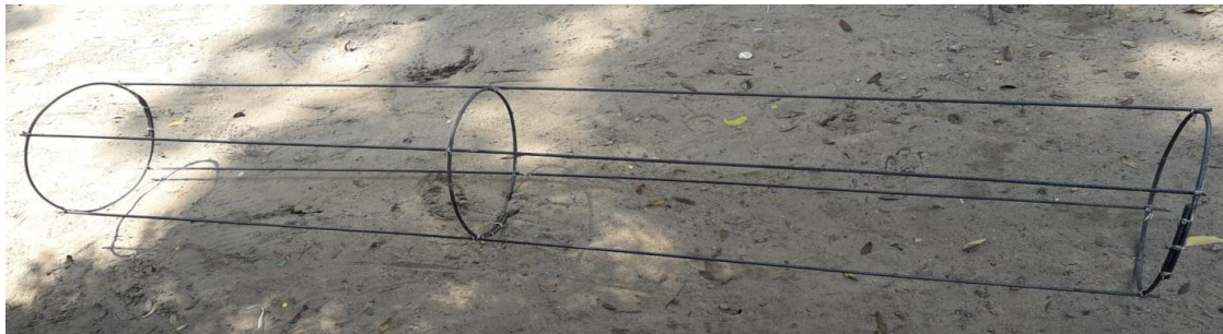
Fig.1 Reinforcement of Pipe
