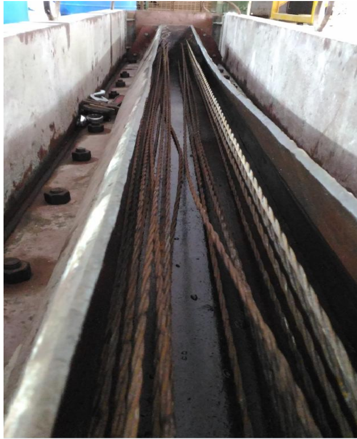
Fig. 3 Before pre tension of Strands
