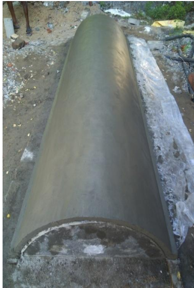
Fig.3 Finished shape of ferropolymer Channel
