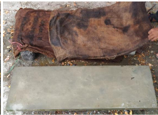
Fig.25 Covering with Gunny Bag
