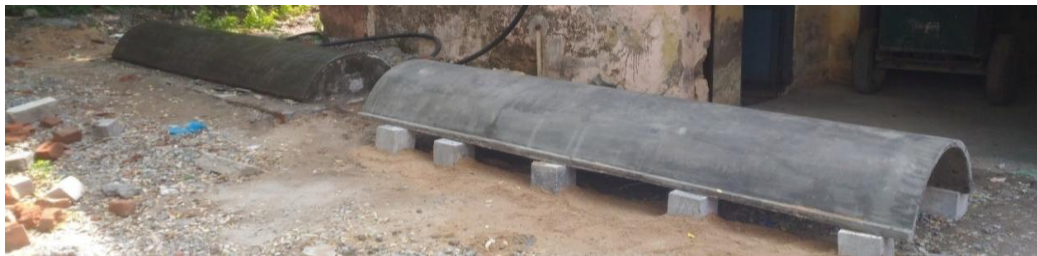
Fig.4 Ferropolymer Channel After Removing from the Mould
