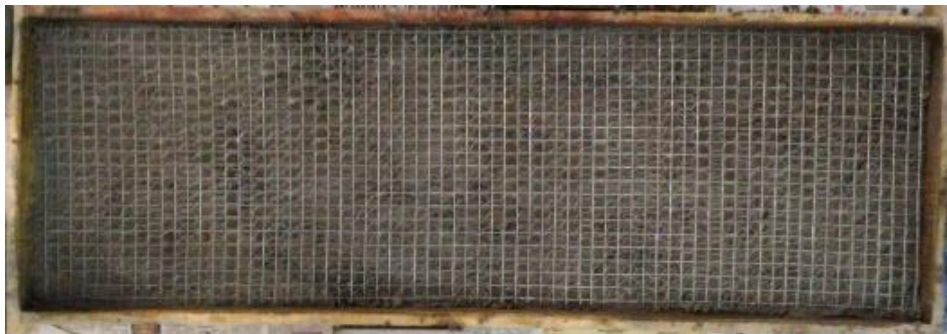
Fig.18 Placing of D type Mesh
