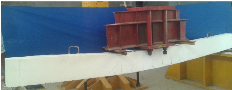
Fig.12 Failure of Beam at Ultimate Load GB2
