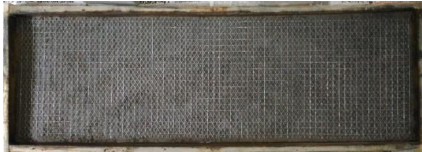
Fig.12 Placing of C Type Mesh
