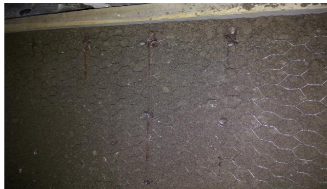
Fig.14 Mortaring on Skletal Steel
