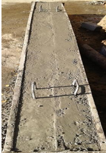
Fig. 4 Casting of Geopolymer Concrete Beams
