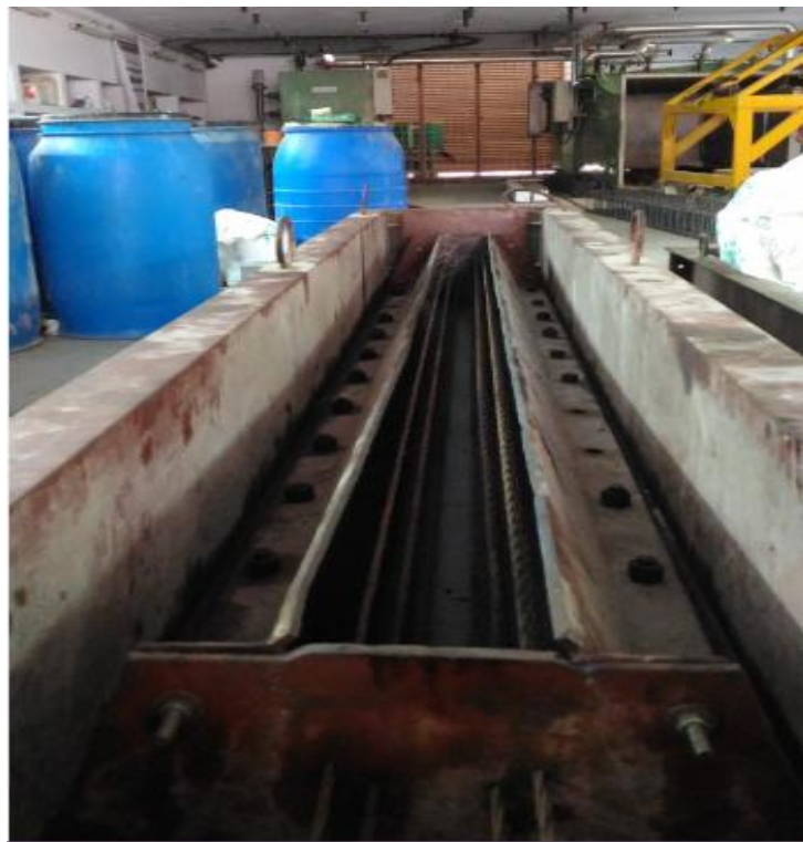
Fig.4 After pre tensioning of Strand
