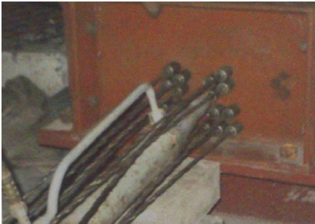
Fig.2 Pre tensioning of Strands
