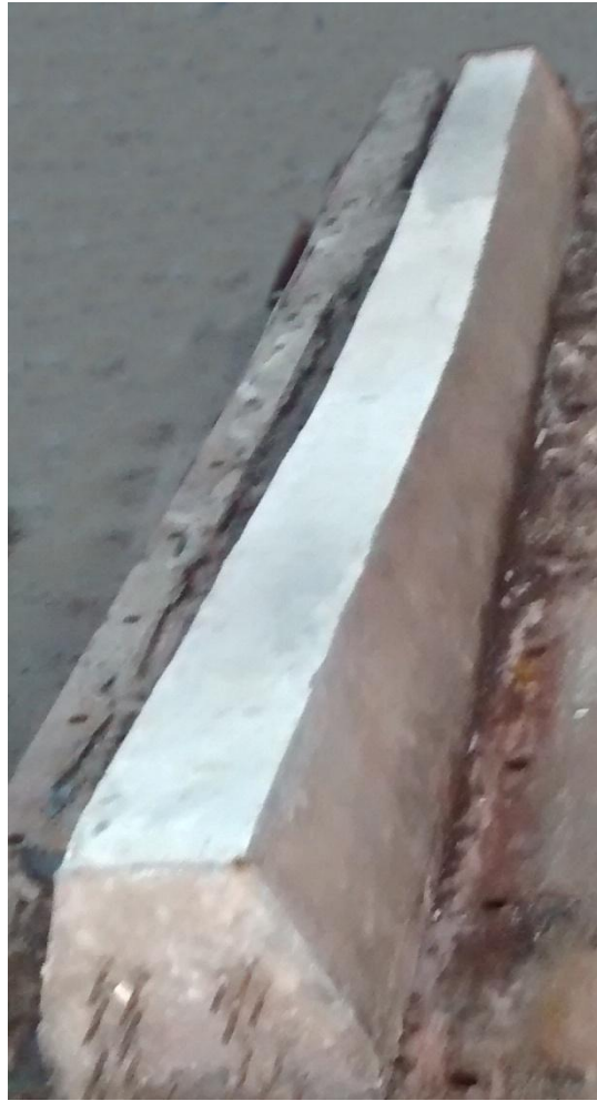
Fig.8 Ambient curing of GPC Sleeper
