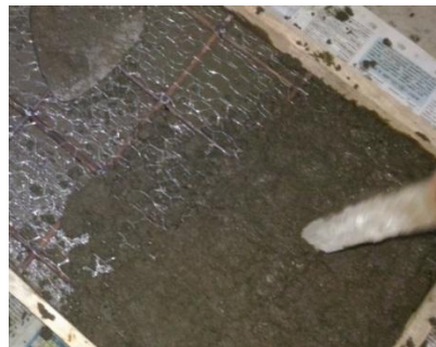
Fig.9 Applying Cement Mortar and Compaction
