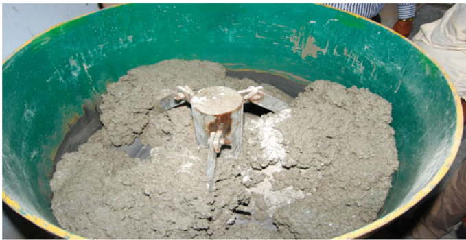
Fig. 3 Mixing of geopolymer concrete
