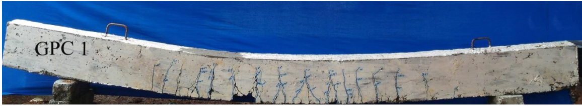
Fig. 7 Crack Pattern of GPC1
