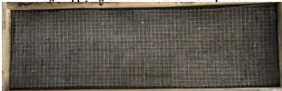
Fig.10 Placing of Mesh Layer
