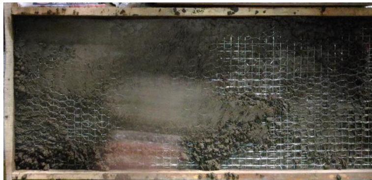
Fig.17 Applying of Mortar
