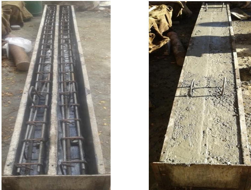
Fig.3 Casting of Conventional Concrete Beams
