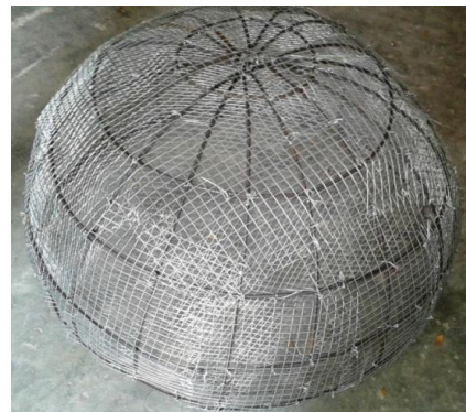
Fig. 6 Mesh on reinforcement
