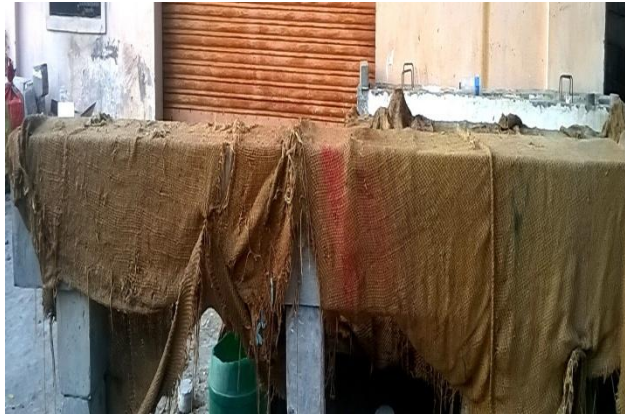
Fig.6 Curing of Ferrocement Box Beams
