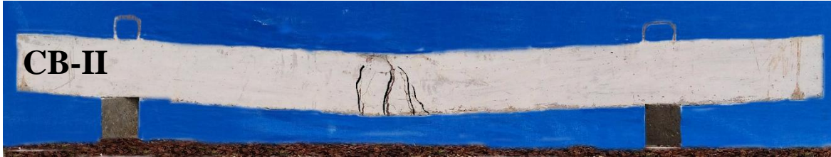
Figure 25 Cracking Pattern of Control beam Under Cyclic loading
