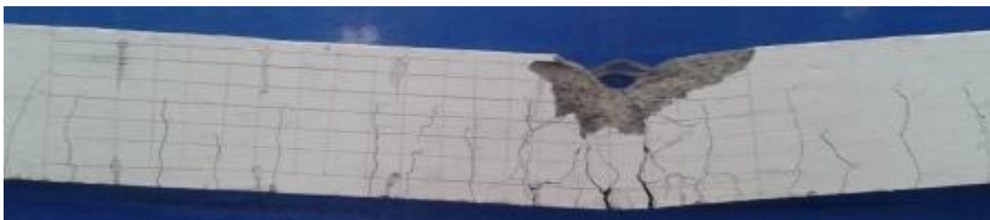
Fig.7 Crack Pattern of CB1
