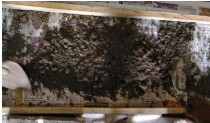
Fig.20 Placing Bottom Cover Mortar
