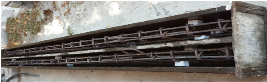
Fig. 7 Reinforcement grills for beams
