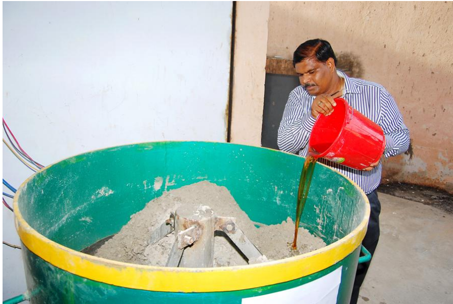
d.Mixing of Raw Materials in Pan Mixer
