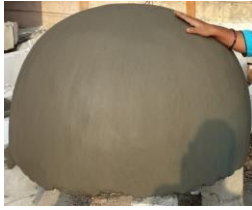
Fig. 8 Outer surface of Dome
