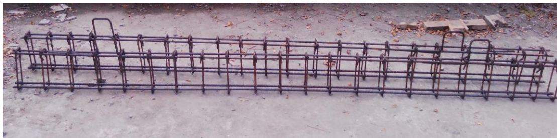
Figure 15 Reinforcement Grill for Beams
