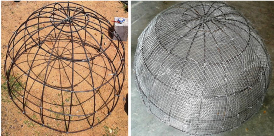
Fig. 23 Dome reinforcement
