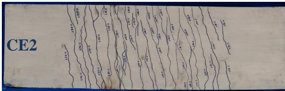
Fig.33 Crack Pattern of CE2
