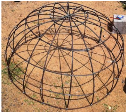
Fig. 5 Dome reinforcement
