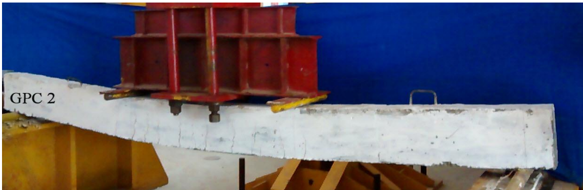
Fig. 11 Failure of Beam at Ultimate Load (GPC2)
