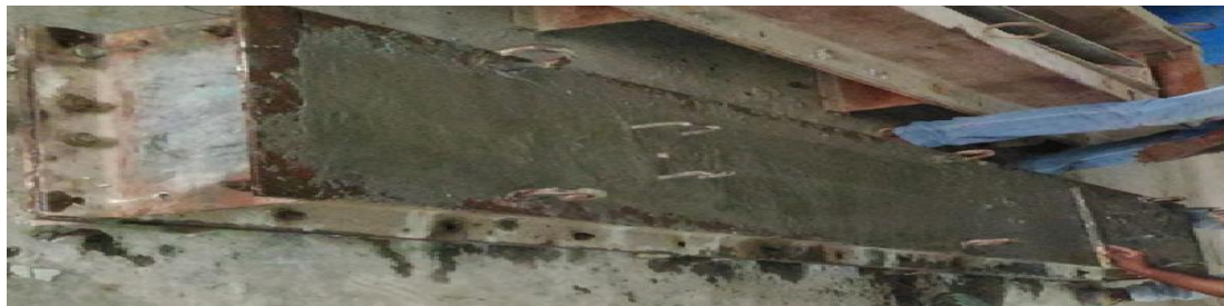
Figure 16 Casting of Beams
