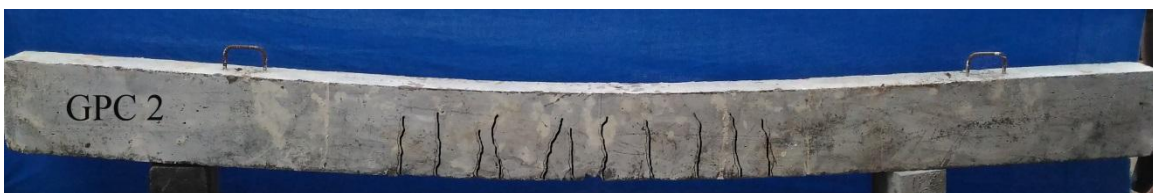
Fig. 13 Crack Pattern of GPC2
