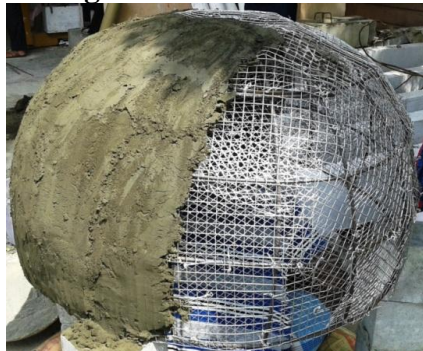
Fig. 7 Application of mortar
