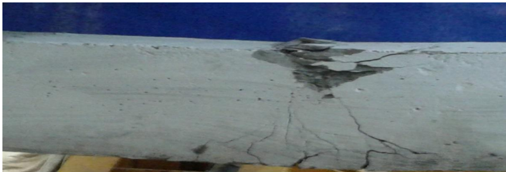
Fig.13 Crack pattern of CB2
