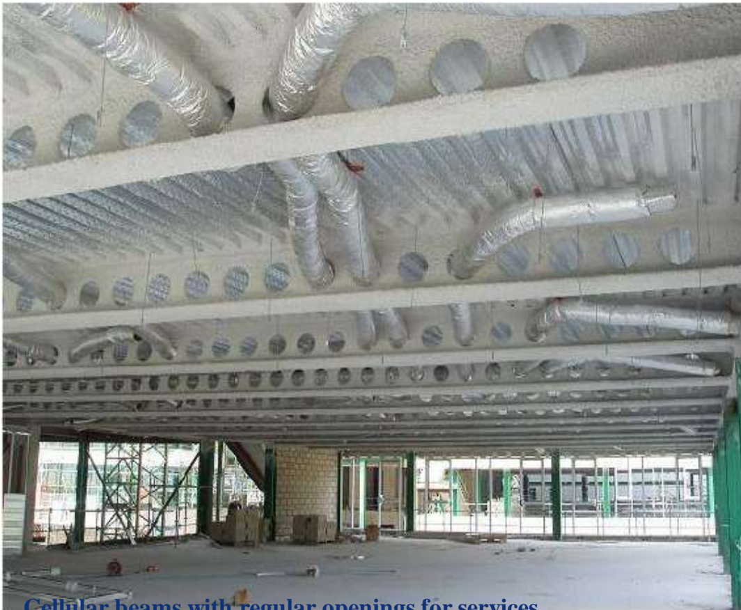
Cellular beams with regular openings for services
